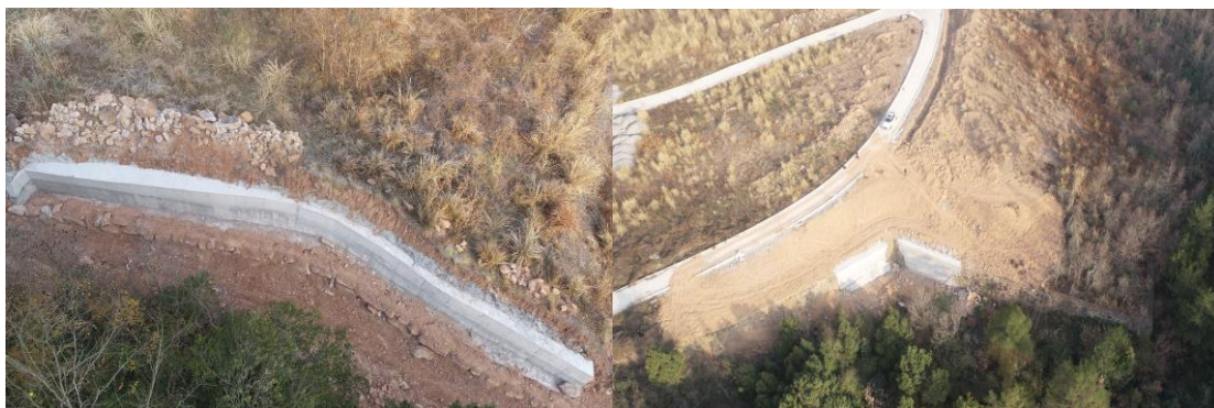
1#渣场 C20 挡墙修复 (2023.11)
